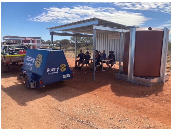
Two recently constructed shelters on the Stuart Highway at the Indulkana Bus Stop.
