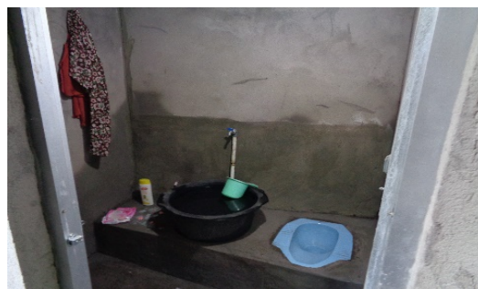
Using as a bathroom they plumbed it to their water supply
